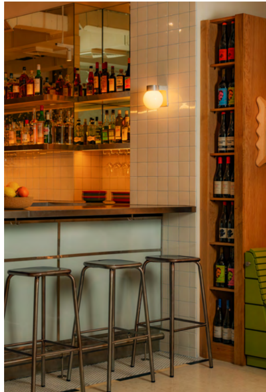
Wall Coverings, Front Desk and other millworks manufactured combining wood veneer and solid wood. Counter bar manufactured with the combination of HPL and Stainless Steel. Service Island manufactured with a combination of HPL, Stainless steel and tempered glass.
